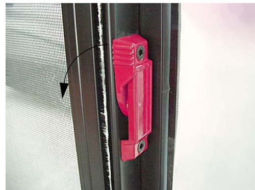
Pull latch outward to slide window open
