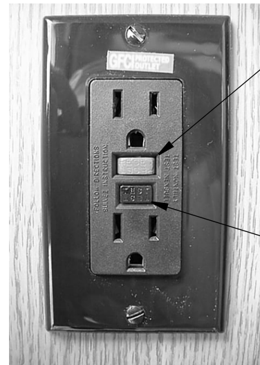
GFCI Outlet (Ground Fault Protector)
