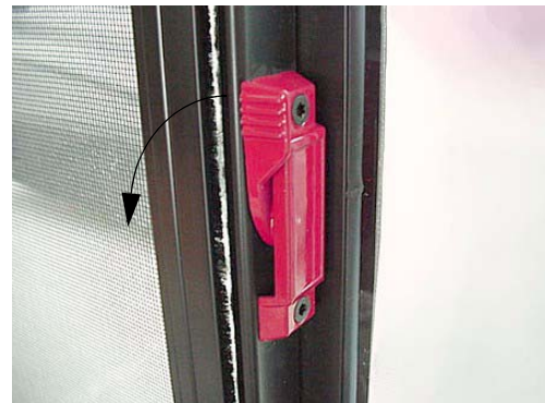
Pull latch outward to slide window open
