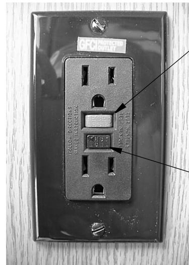
GFCI Outlet (Ground Fault Protector)
