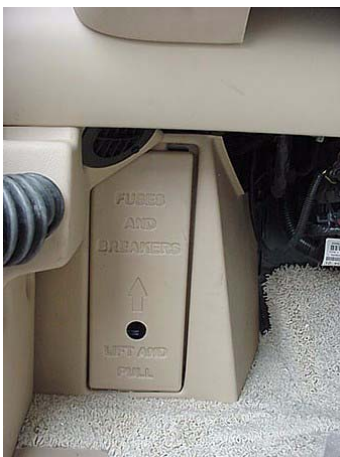
Automotive Fuse/Breaker Panel (beneath left end of dash)
