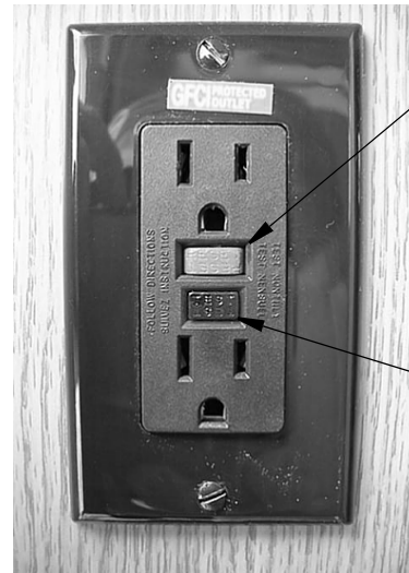
GFCI Outlet (Ground Fault Protector)
