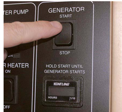
Generator Switch and Hourmeter
