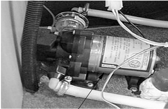
Water Pump (typical)
