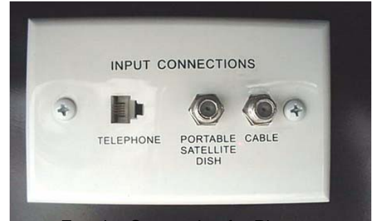
Exterior Connection for Phone, Satellite Dishes and Cable TV (In Water Center or Shoreline Compartment)
