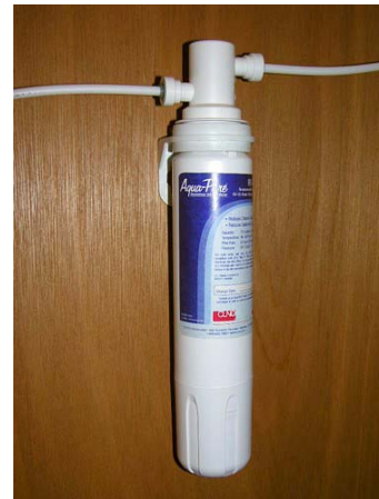
Water Filter Assembly (Located below galley sink) * Typical View - your coach may vary
