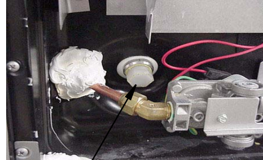
Water Heater Drain Plug (Remove with socket)
