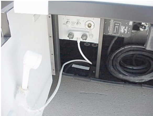
Water Service Center
