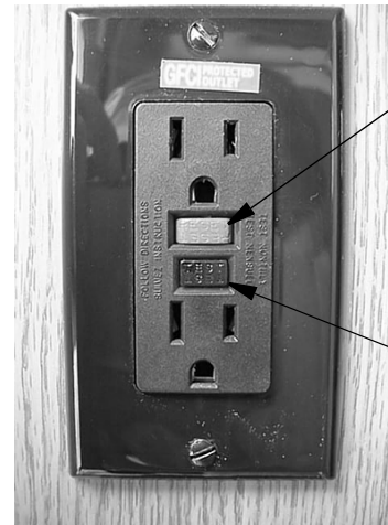
GFCI Outlet (Ground Fault Protector)
