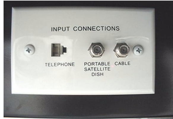
Exterior Connection for Satellite Dish and Cable TV (In Water Center or Shoreline Compartment)
