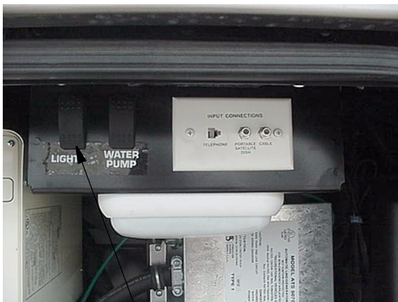
Utility Light Switch
