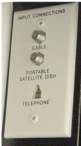
Exterior Connection for Satellite Dishes and Cable TV (In Water Center Compartment)
