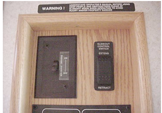
Electric Water Heater Switch above OnePlace panel
