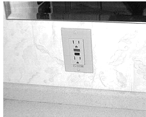
Ground Fault Circuit Interrupter (GFCI)
