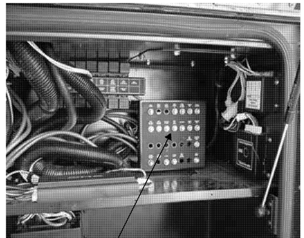
Automotive 12-Volt Breaker Panel
