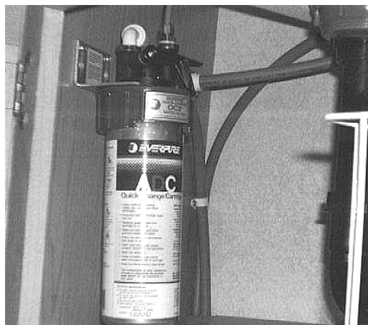
Water Filter Assembly - Below Galley Sink
