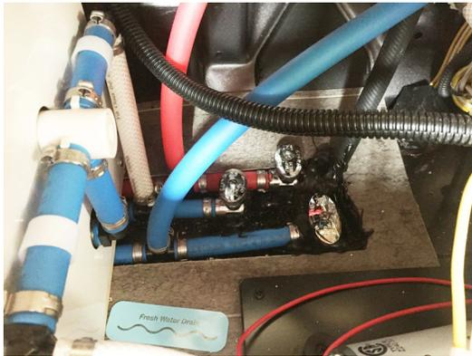
Waterlines and Tank Drain Valves
