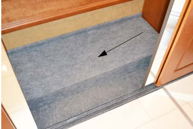
Access Panel (Located on bathroom wardrobe floor)
