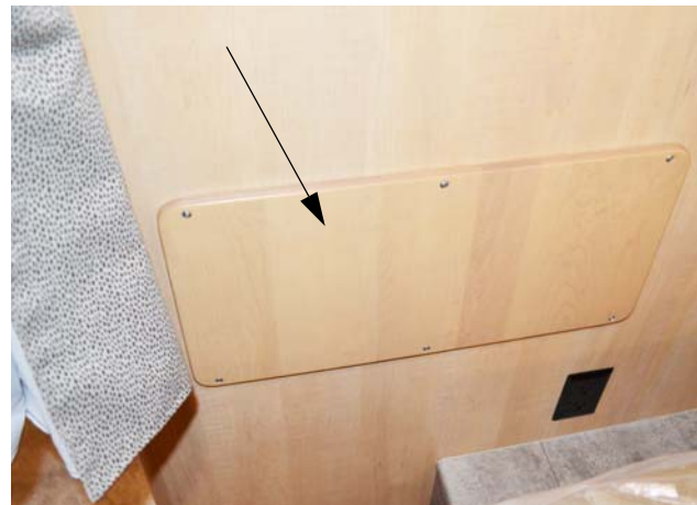
Refrigerator Access Panel (Located on front bedroom wall) *Model 23T
