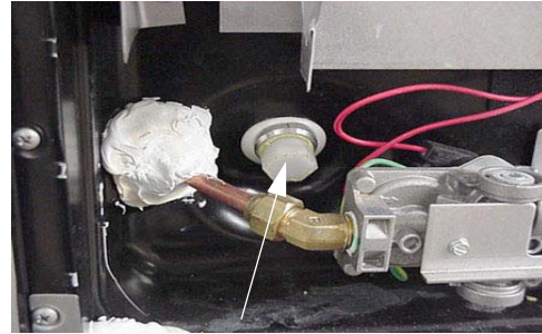
Water Heater Drain Plug (Remove with socket)
