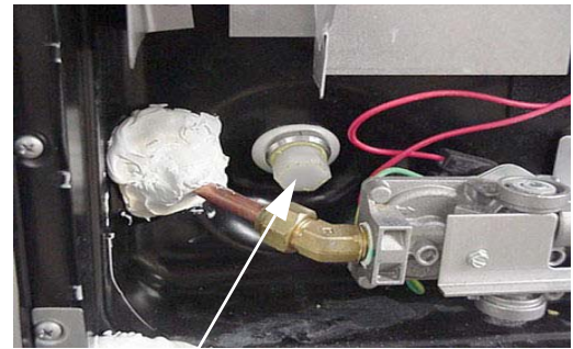
Water Heater Drain Plug (Remove with socket)
