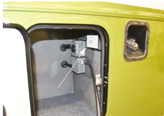
Cable TV Connection (Located in an exterior driver side compartment) -Typical installation shown
