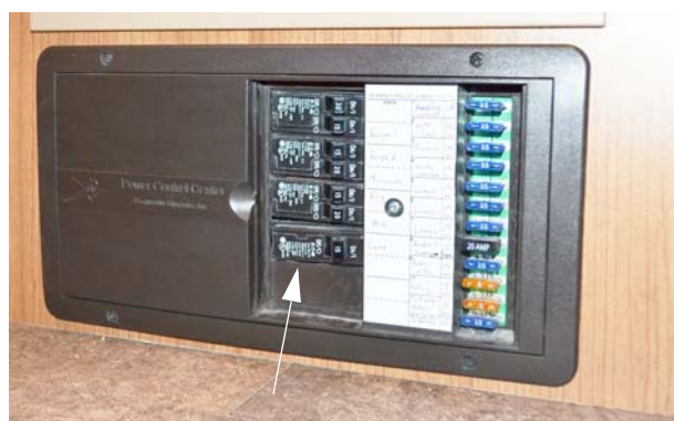
120-Volt House Circuit Breakers -Typical View
