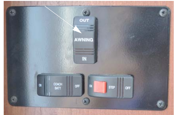
Power Awning Switch (Located near entrance door)
