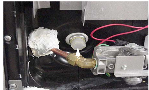
Water Heater Drain Plug (Remove with socket) -Typical View
