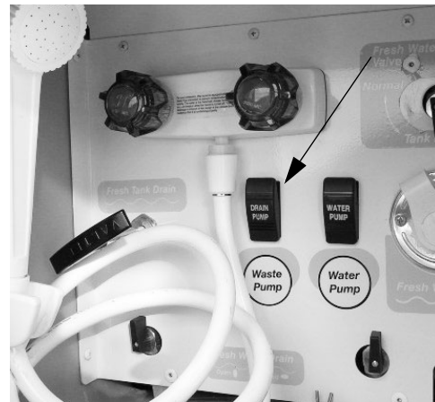
Waste Pump Switch (Located in water service center) -Typical View
