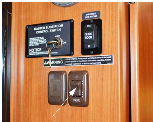
Main Tank Valve Switch (Located near monitor panel area) -Typical View
