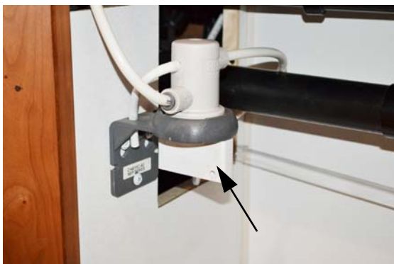
Diverter Plug (installed in filter socket)
