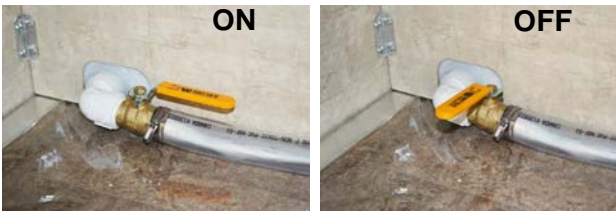
Water Tank Drain Valves *Model 24M shown
