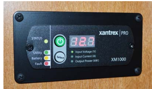
Inverter Control Panel (Located near monitor panel) -Typical View
