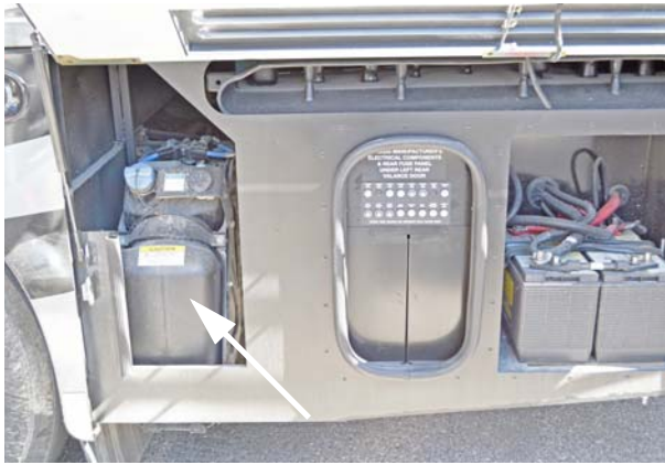
Diesel Exhaust Fluid Fill Tank (Located in driver side compartment behind the rear wheel) -Typical View
