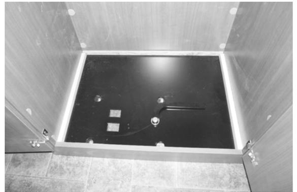
3. Rotate the Locking Arm fully **CLOCKWISE** to the **locked** position, securing the Wardrobe Cabinet to the floor plate.
