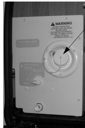
Water Tank Gravity Fill
