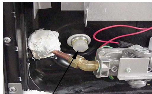
Water Heater Drain Plug (Remove with socket)
