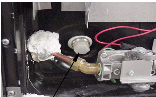
Water Heater Drain Plug (Remove with socket)
