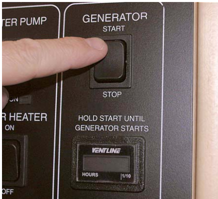
Generator Switch and Hourmeter on monitor panel
