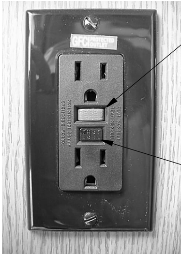
GFCI Outlet (Ground Fault Protector)
