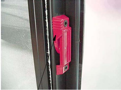
Pull latch outward to slide window open
