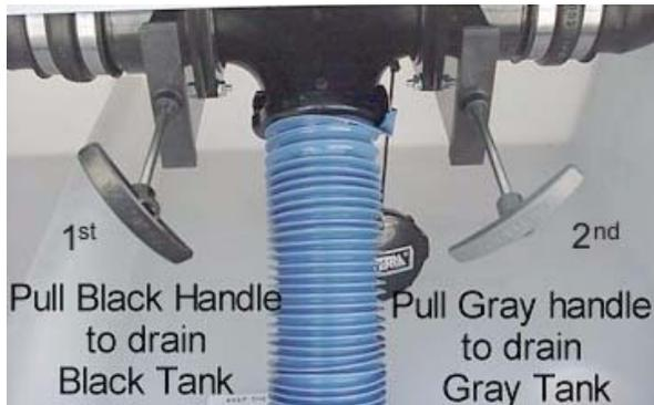
Holding Tank Dump Valves (Typical)
