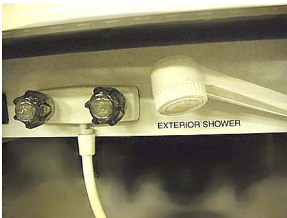
Exterior Shower/Wash Station (Typical)
