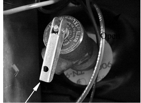
Lift handle straight out to open P-T valve when water heater is cold *
