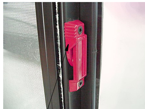
Pull latch outward to slide window open
