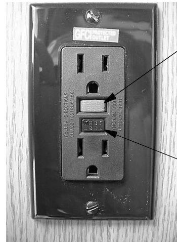
GFCI Outlet (Ground Fault Protector)
