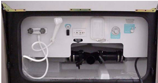
Water Service Center
