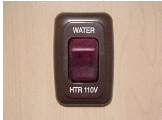
Electric Water Heater Switch (Typical)
