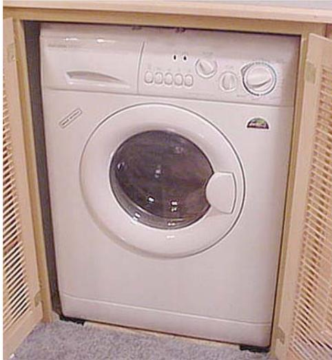
The washing machine water supply faucets are located inside the cabinet door above the machine. Always turn supply faucets off when not using washing machine to avoid possible water leaks if a hose or hose gasket should fail.
