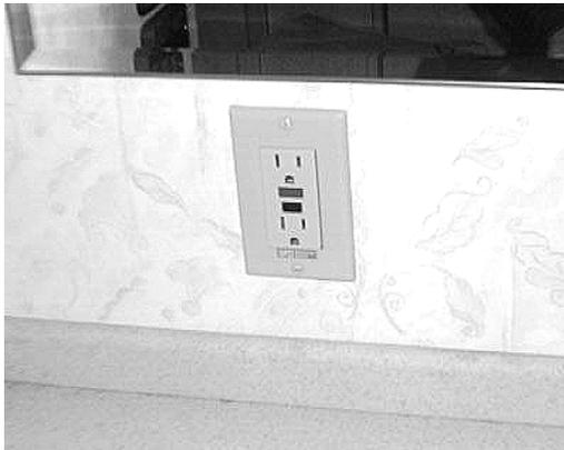
Ground Fault Circuit Interrupter (GFCI)
