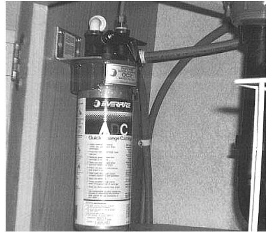
Water Filter Assembly - Below Galley Sink
