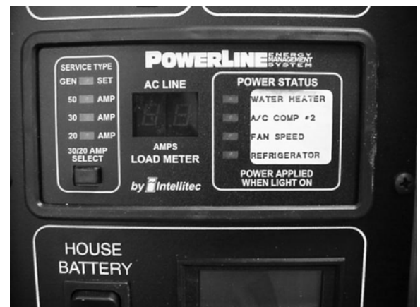
EMS Display on OnePlace Monitor Panel
