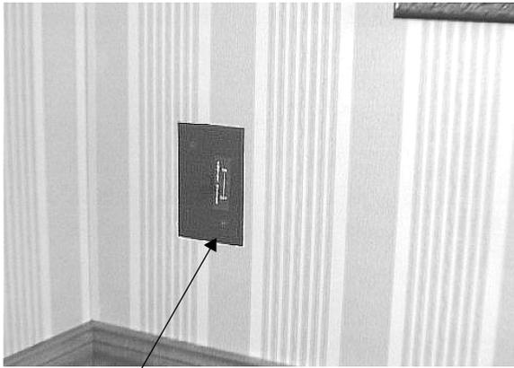
Engine Block Heater Switch
