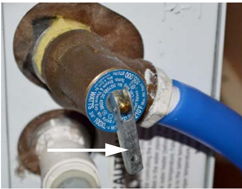
Pressure Temperature Relief Valve (Lift handle only when water heater is cold)
