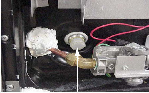
Water Heater Drain Plug (Remove with socket)
