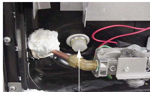
Water Heater Drain Plug (Remove with socket)
