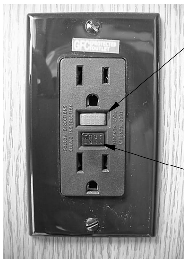
GFCI Outlet (Ground Fault Protector)
