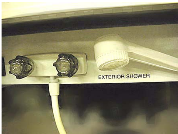
Exterior Shower/Wash Station -Typical View
