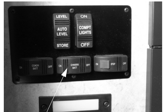
Chassis Battery Disconnect Switch (Located inside the entrance door)
