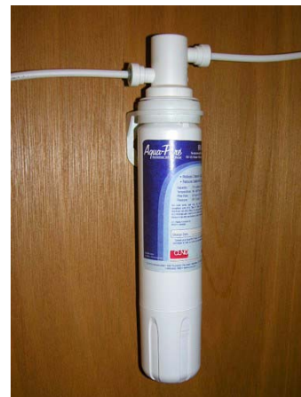
Water Filter Assembly below Galley Sink
